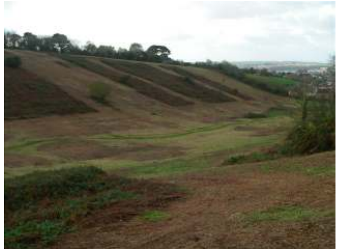
Strips being cleared for access and planting
